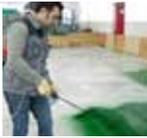
**BETON COLOR DYE:** Concentrate powder colours to be dilute in 4 lt of Acetone to colour concrete floors. The BETON COLOR above showed colours are indicative. They are not RAL because they are not varnish but the result of a chemical reaction with the concrete. As a result the tonality can change according with the kind of concrete. We recommend to make a preliminary test to be sure of the colour reached.
